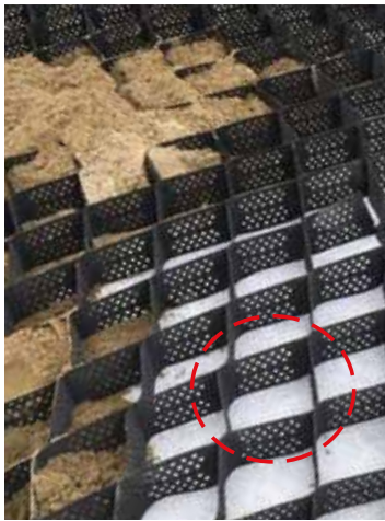
SLOPE EROSION CONTROL by ENVIRO GRID™
